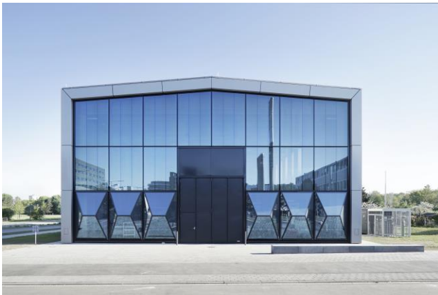
Figure 7: ETA-Factory in Darmstadt (Image source: PTW, TU Darmstadt / Eibe Sönnecken)
