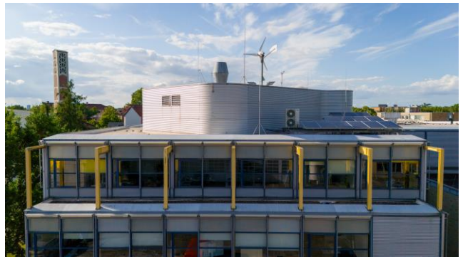
Figure 9: Infrastructure for self-sufficient electricity supply using wind turbines and photovoltaic systems for the learning factory at the IWF of the Technische Universität Braunschweig (Image source: IWF TU Braunschweig)
